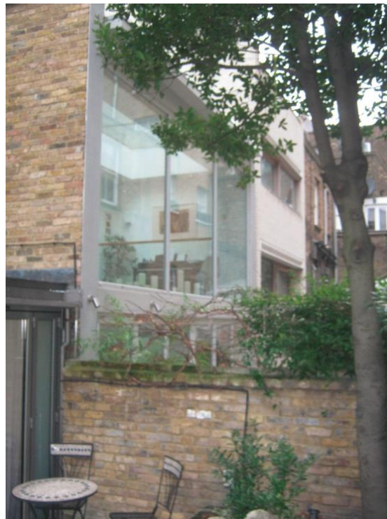
Front elevation (No.14 to left of photograph) (top) and rear elevation as seen from No.12 (bottom).
